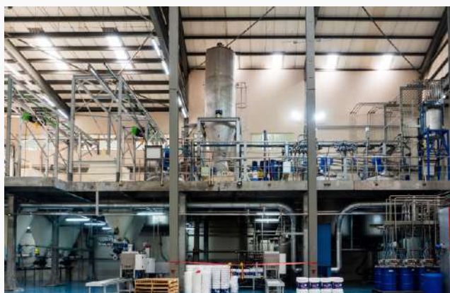
Picture of Newly Commissioned Ultramodern Berger Paints Factory
